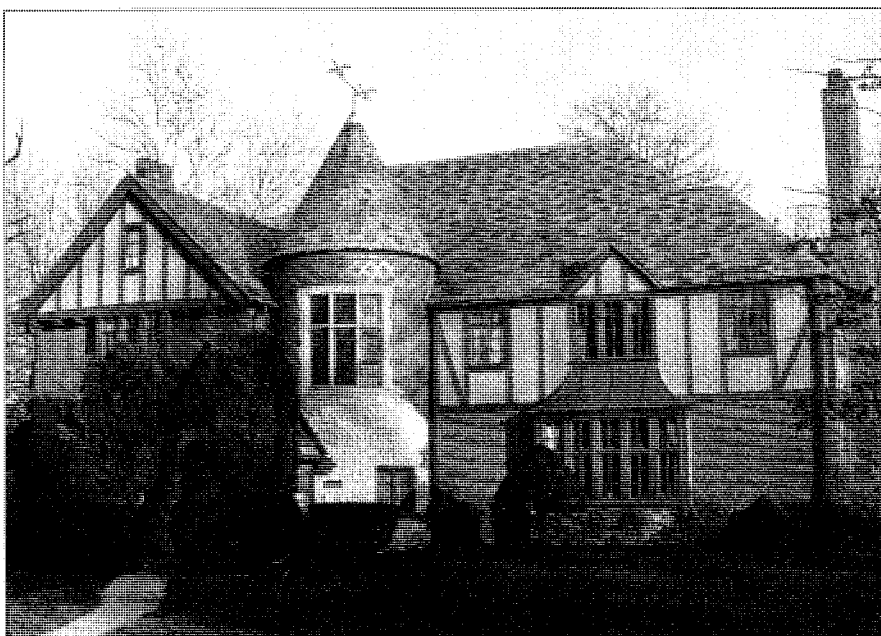
French Colonial/Norman Revival , Elmer McKesson House, Toledo, 1933
